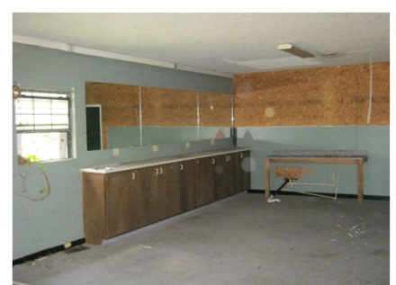
Partial interior of out building
