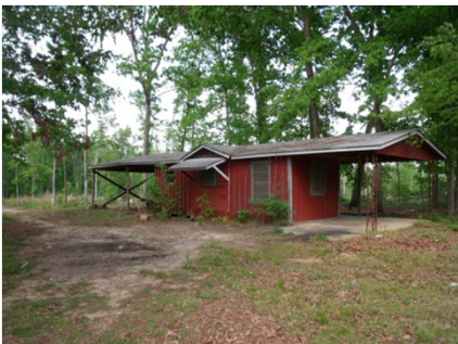
Workshop w/ tractor shed
